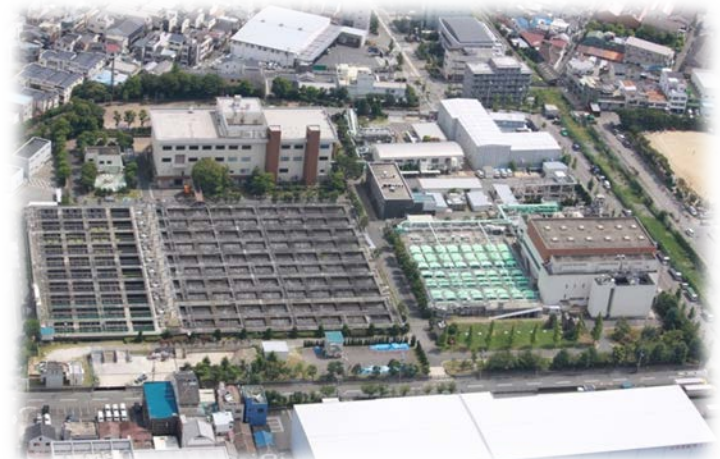
Waste water treatment
